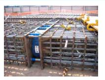
O-cells are installed within the barrette reinforcement
